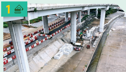
1 於松嶺路附近建造臨時工作台 Construction of temporary working platform near Chung Ling Road
