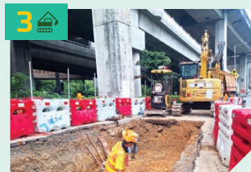
3 於文林路附近進行地下設施勘探 Underground utilities investigation near Man Lam Road
