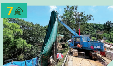
7 獅子山隧道公路近曾大屋進行鋼管樁工程，以配合支路建造工程 Installation of pipe piles near Sha Tin Tau Village at Lion Rock Tunnel Road near Tsang Tai Uk for the construction of slip road
