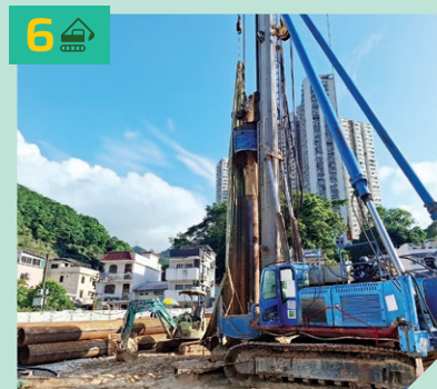
6 於沙田頭村安裝臨時支架，配合興建地下行車道 Installation of temporary supports at Sha Tin Tau Village to facilitate the construction of underpass
