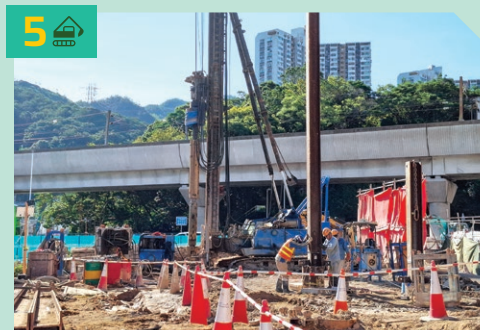
5 於獅子山隧道公路與大涌橋路交界工地進行鋼管樁工程 Pile piling at the works sites at the junction of Tai Chung Kiu Road and Lion Rock Tunnel Road
