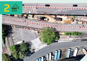
2 於成運路附近進行鑽孔樁工程，以興建高架橋 Bored piling works near Shing Wan Road for the construction of viaduct
